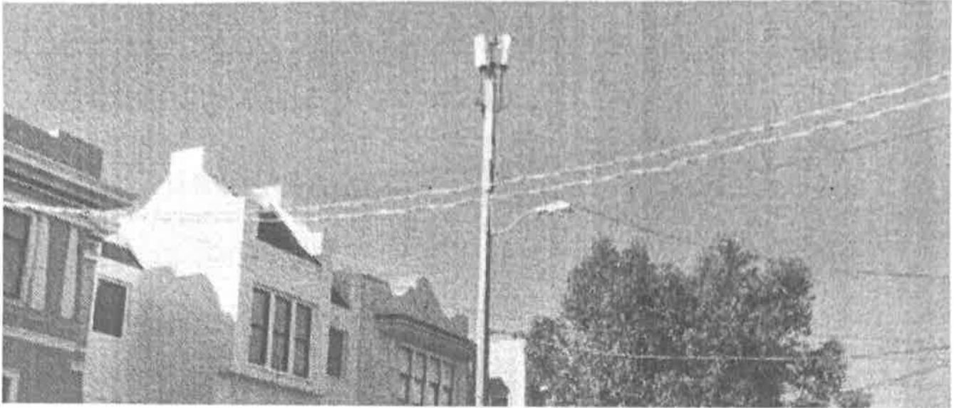
TOP: Disfavored use of multiple panel antennas with wide offset mechanical tilt brackets (evaluate electronic tilt alternatives) and loose cabling
