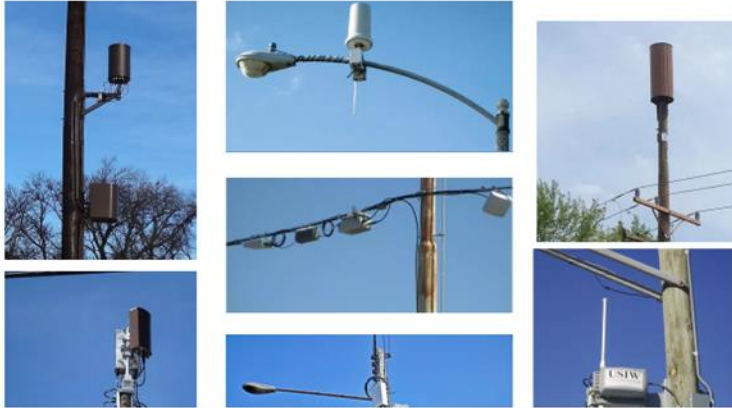
Examples of 5G Small Cell Installations
