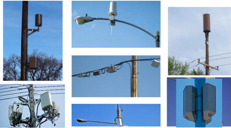
Examples of 5G Small Cell Installations
